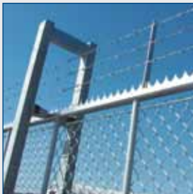
Serrated anti-climb top rail
